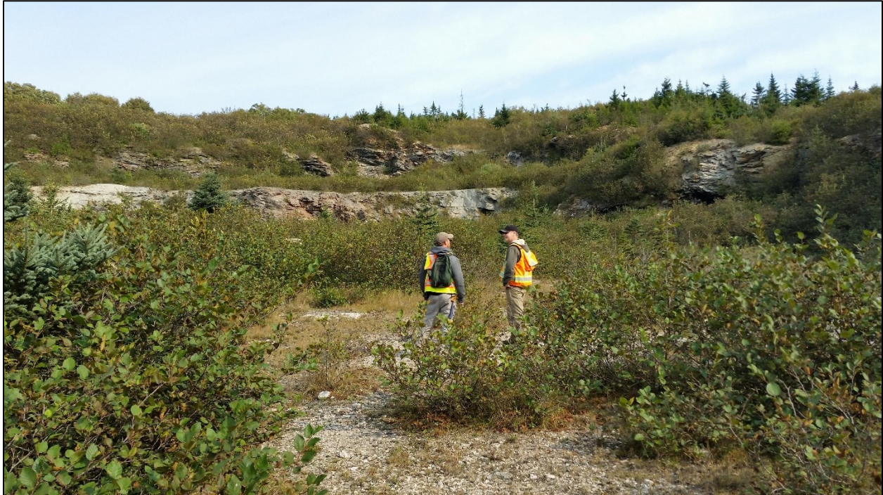
Figure 12.5: Current Vegetation and Face Exposures in the Cape Spencer Open Pit Uppermost Excavation
